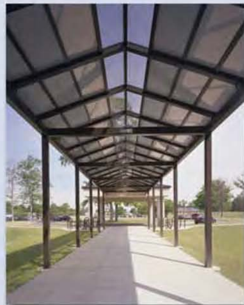
Transportation Inn • Building 1750 Fort Eustis, Virginia Architect: DJG, Inc.
