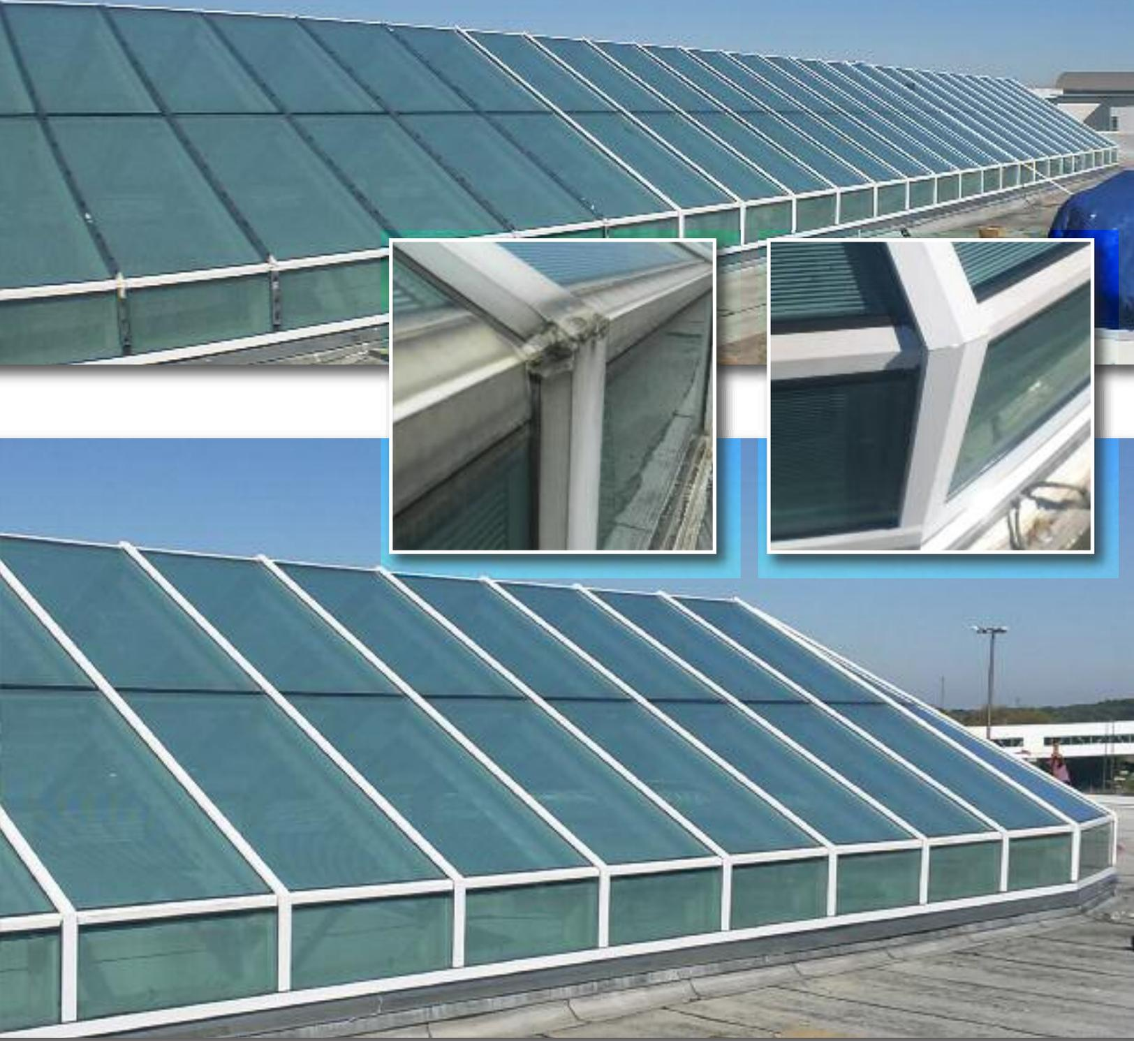
Existing ridge skylights, on three separate terminals, were renovated by replacing the caps, flashing and caulking. During Super Sky's in-depth inspection, the glass was determined to be intact and did not require replacement.
