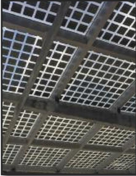
Building Integrated Photovoltaics (BIPV) systems consist of integrating photovoltaics modules into a skylight system. While simultaneously serving as building envelope material and power generator, BIPV systems can provide savings in materials and electrical costs, reduce use of fossil fuels and emission of ozone depleting gases, and add architectural aesthetics to any building.
