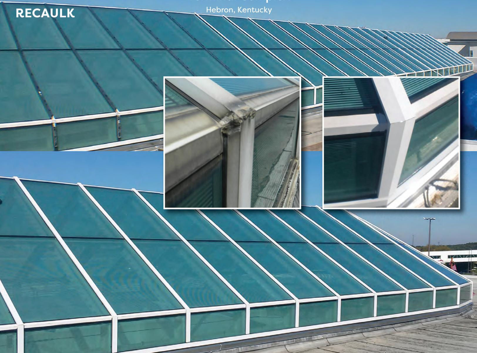
Three existing ridge skylights, on three separate terminals, were renovated by replacing the caps, flashing and caulking. During Super Sky's in-depth inspection, the glass was determined to be intact and did not require replacement.
