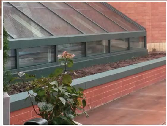
The existing skylight over the main atrium of the hotel entrance was reglazed by Super Sky to eliminate leakage problems, as well as improve the aesthetic appearance of the area. The existing skylight and side lites had seal failures that left the glass lites fogged and opaque.
