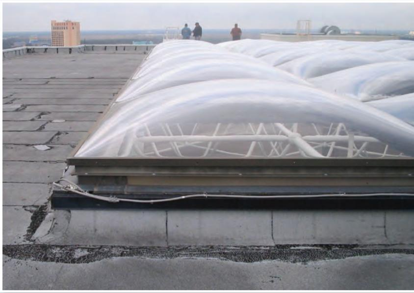
Existing acrylic multiple dome skylights on a gutter system, supported by a steel space frame were removed and replaced by Super Sky to eliminate leakage problems, and update with a state-of-the-art structure.
