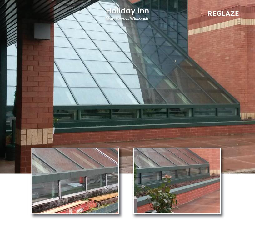
The existing skylight over the main atrium of the hotel entrance was reglazed by Super Sky to eliminate leakage problems, as well as improve the aesthetic appearance of the area. The existing skylight and side lites had seal failures that left the glass lites fogged and opaque.
