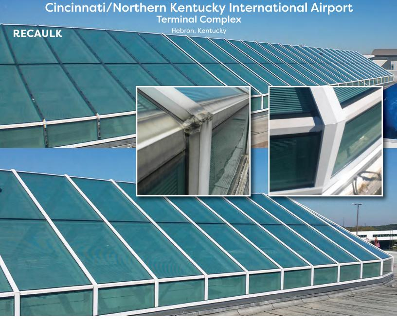
Three existing ridge skylights, on three separate terminals, were renovated by replacing the caps, flashing and caulking. During Super Sky's in-depth inspection, the glass was determined to be intact and did not require replacement.
